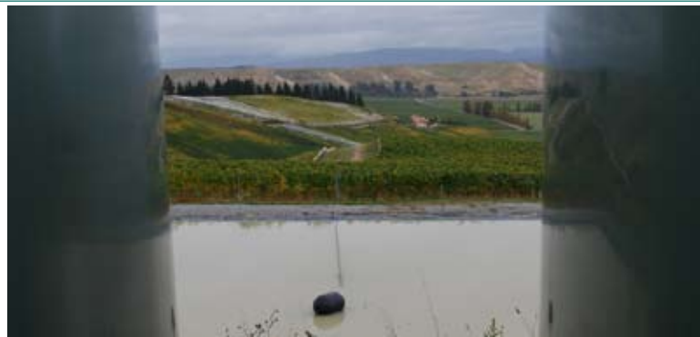
The Nautilus Clay Hills dam, framed by two water storage tanks, provides insurance against water restrictions being applied.
